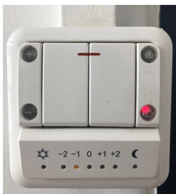
Figure 2.20 – Control box for electric lighting and temperature set point (Siemens UP 231/2). The left switch (+/-) is used to select the desired temperature set point, indicated at the bottom of the switch.
