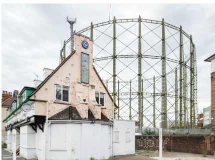
Kennington Gasholder Station
