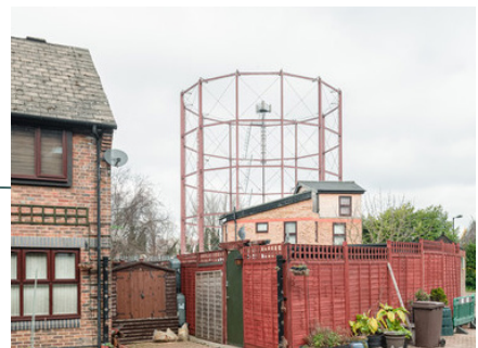
Rotherhithe Gasholder Station
