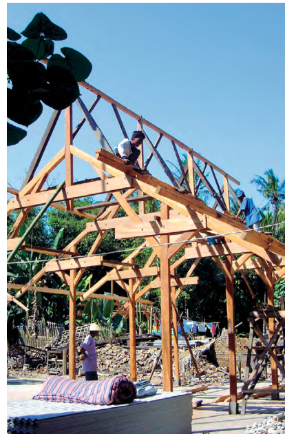
Construction de la structure en bois, 2010 © Aga Khan Award for Architecture
