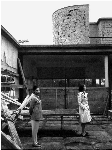
Fig.57 Construction de la villa Savoye, ca. 1928, Poissy
