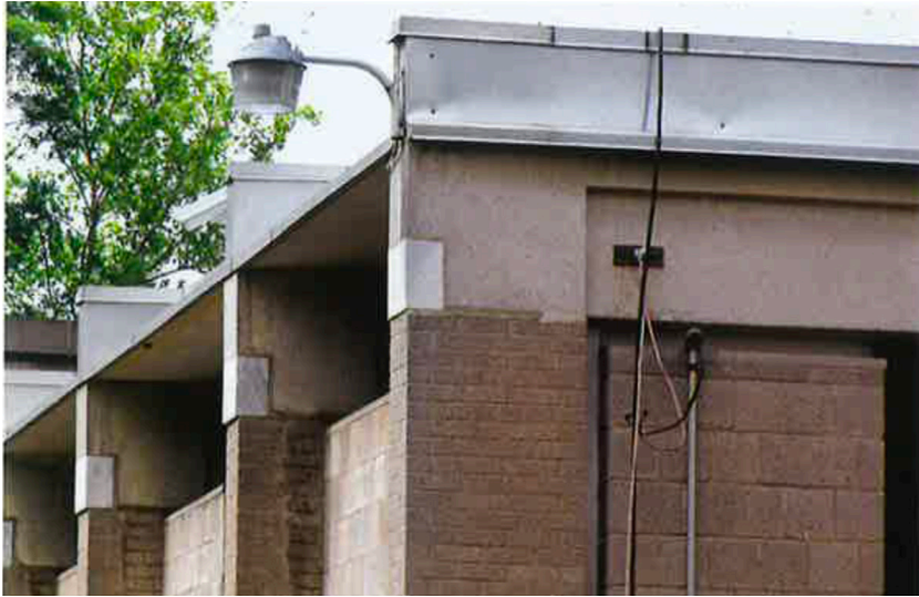
Fig.22 Les «bouchons» de marbre. Louis Kahn, Tribune Review Building, 1962, Greensburg
