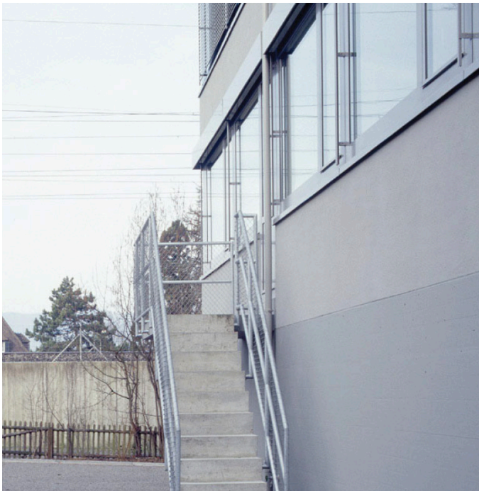
Studio House, Zollikon, 1998-2001 Architectes: Christ & Gantenbein
