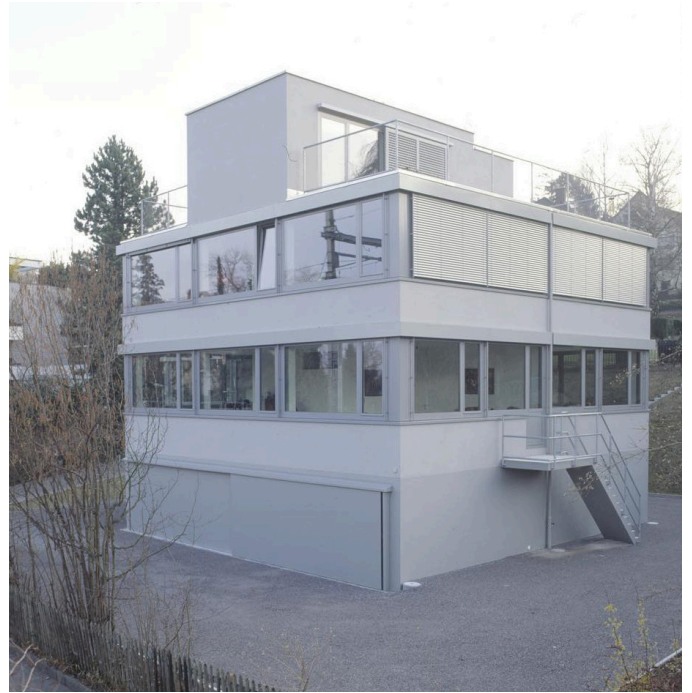
Studio House, Zollikon, 1998-2001 Architectes: Christ & Gantenbein
