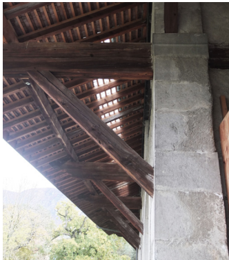
Fig. 18: Tuiles translucides [Allémann 2020]
