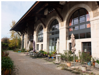
Fig. 32: Façade sud [Allémann 2020]
