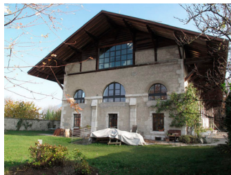
Fig. 13: Façade ouest [atba architecture]
