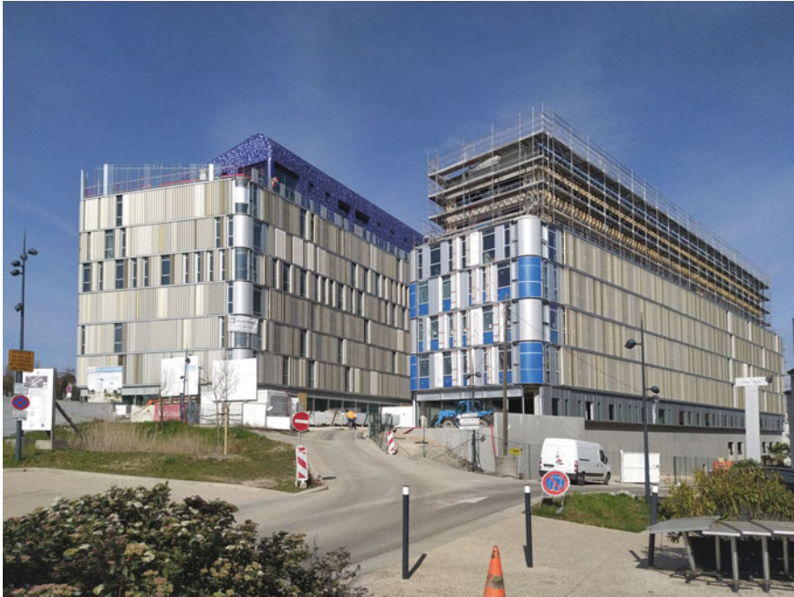
Fig. 10.9 New tertiary centre under construction (photo: Ville de Besançon, 2021)
