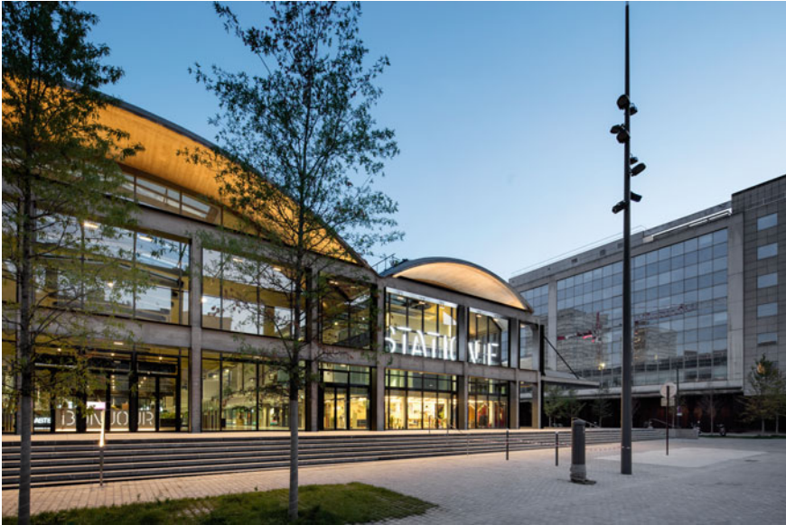
Fig. 2.4 Station F, Paris (FR). Transformation of the former Halle Freyssinet of Gare d'Austerlitz into a start-up campus. Wilmotte & Associés SAS, 2017 (photo: Patrick Tourneboeuf, 2017)
