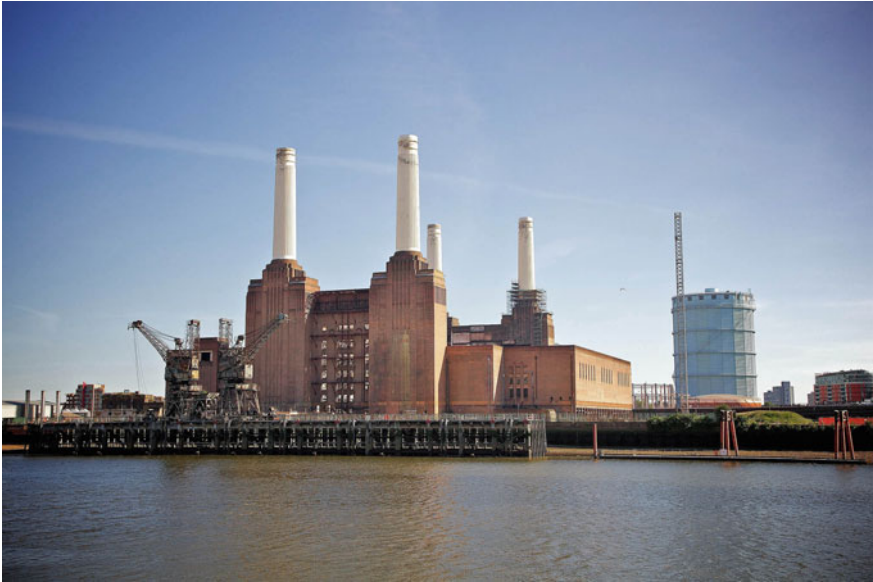
Fig. 2.17 Battersea Power Station, London (UK). Transformation of a former power station into a headquarters in the heart of a 7.6-ha new development. Masterplan by Rafael Viñoly Architects, ongoing project (photo: Aurelien Guichard, 2010)
