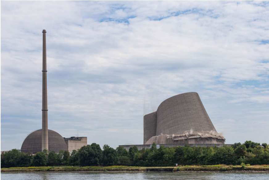
Fig. 2.16 Mülheim-Kärlich nuclear power plant, Mülheim-Kärlich (DE). Collapsed of the cooling tower of the decommissioned nuclear power plant in 2019 (photo: Phantom3Pix, 2019)
