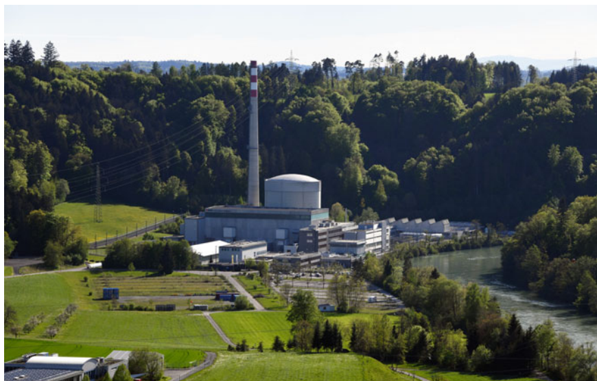
Fig. 2.15 Mühleberg Nuclear Power Plant, Canton of Bern (CH). Decommissioning of buildings as part of the strategy of abandoning nuclear power in Switzerland started in 2020 and to be completed by 2034 (photo: Emmanuel Rey, 2021)
