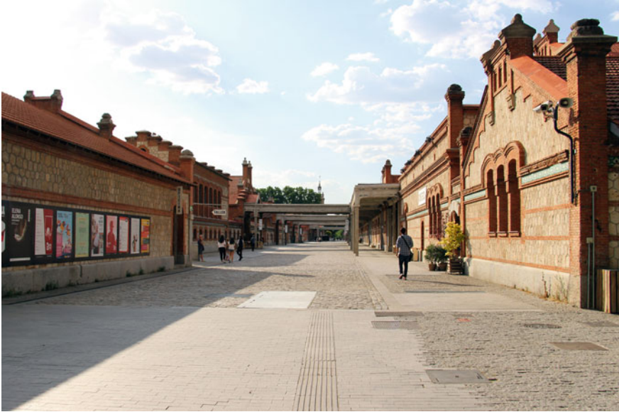
Fig. 2.12 Matadero, Madrid (ES). Regeneration of a former slaughterhouse area into a new neighbourhood dedicated to culture. Ensemble Studio, A. Franco, Martin + Batanero, CH + QS arquitectos, 2006–2012 (photo: Fred Romero, 2017)
