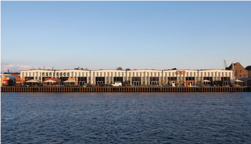
Fig. 2.10 Paper Island, Copenhagen (DK). Rehabilitation of former maritime paper storage facilities into a new district with street food halls, art exhibitions, fashion shows, concerts, and flea markets. Cobe architects, ongoing project (photo: News Øresund – Jenny Andersson, 2016)
