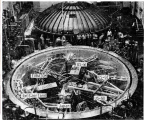
Fig 4: Six LCT coils in the vacuum tank, Oct 1985
