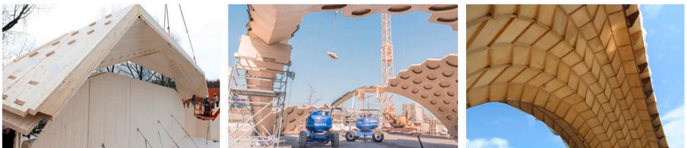
Fig. 1. Three large-scale projects showcasing IATPS (from left to right): The folded structure of the Vidy theater (IBOIS, 2018) [14], the segmented shell of the Buga Wood Pavilion (ICD/ITKE, 2019) [10], the double-layered vault of the Annen head office (IBOIS, 2021) [15].
