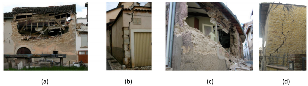
Figure 1. Examples of out-of-plane damage patterns from L'Aquila 2009 earthquake: (a) Out-of-plane mechanism in long walls. (b) Global overturning of external walls. (c) Overturning due to the lack of anchorage between walls and horizontal diaphragms. (d) Corner out-of-plane mechanism [66]. (Sources: Dr. Javier Ortega, Prof. Hugo Rodrigues)
