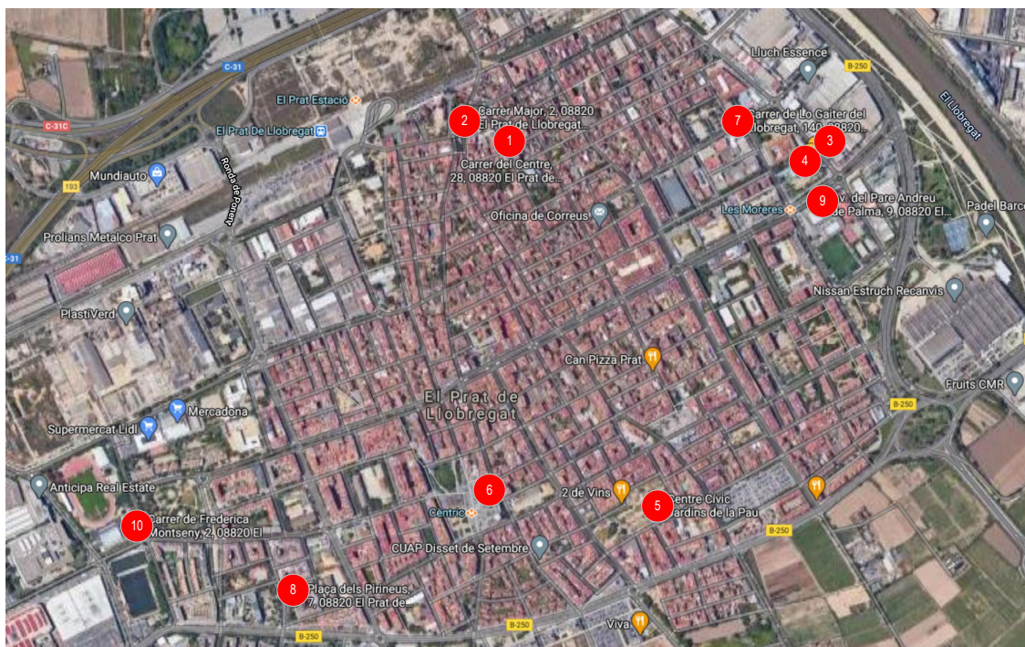
Figure A2. An aerial view of “El Prat del Llobregat” highlighting the locations of the 10 different buildings of the Barcelona demonstration site.
