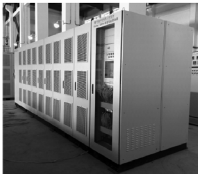
▲ 1MW Solid State Transformer, MMC + DC-DC
