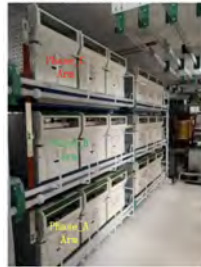
▲ 1.15 MW Solid State Transformer, ISOP AC-DC + DC-DC
