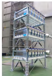
▲ HYOSUNG (left) and LS (right) IGBT-based MMC STATCOMs
