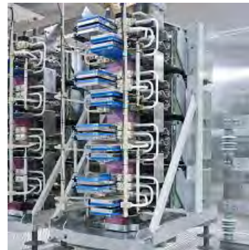
▲ ABB IGBT-based MMC STATCOM
