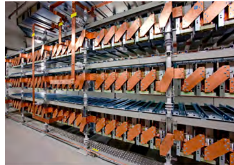
▲ SIEMENS IGBT-based MMC for railway interties (SITRAS PLUS)
