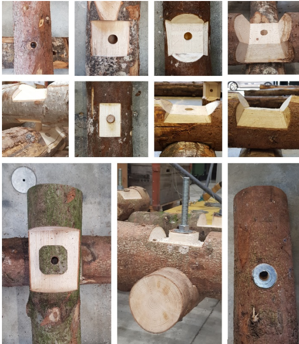
Figure 6: A set of side-side joints with timber and metals fasteners.
