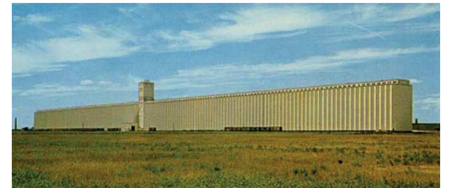
FIG.10 Silo ADM, Hutchinson
