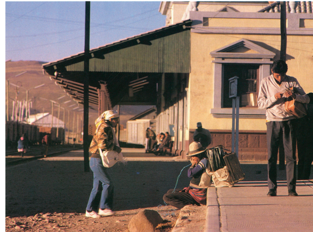
Fig.5 - Train station in Potosí, 1990
