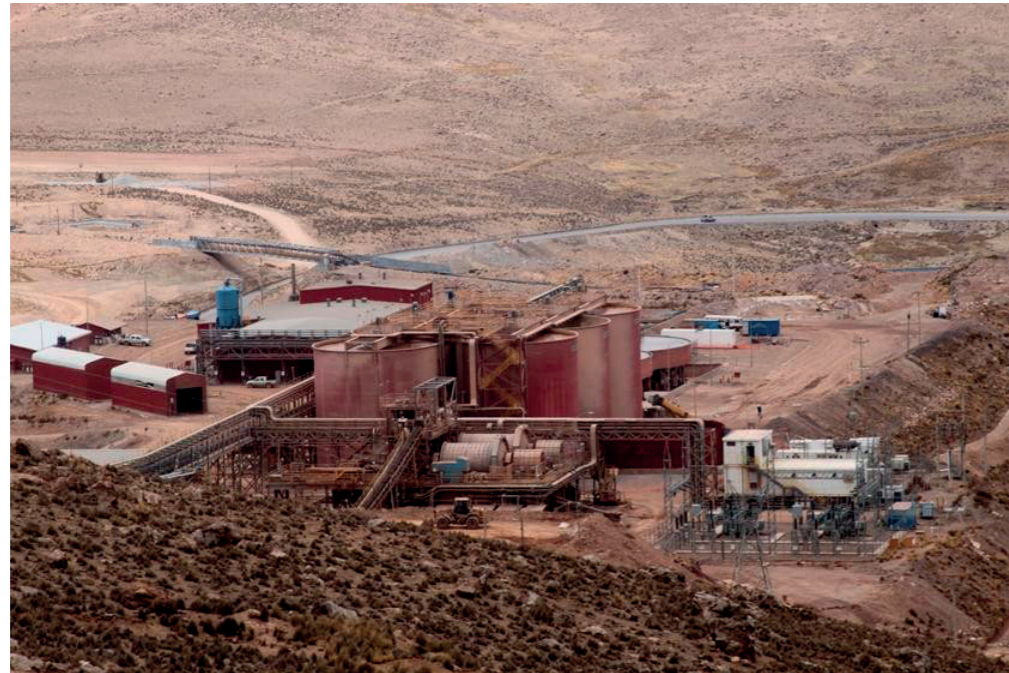
Fig.3- Empresa Minera Manquiri, the tanks are used to store the processing water
