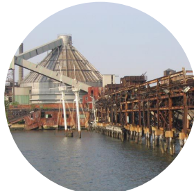
Fig 12: The former Revere Sugar Refinery demolished in 2006
