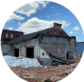
Fig 11: Future sorting and delivery hub for UPS
