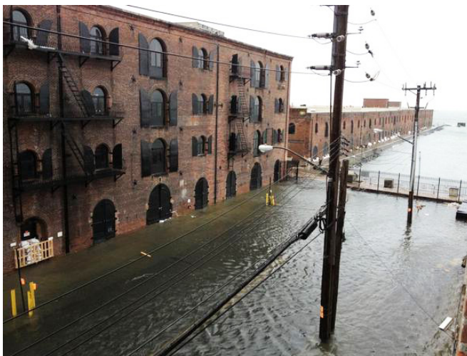
Fig 7: Red Hook after Hurricane Sandy
