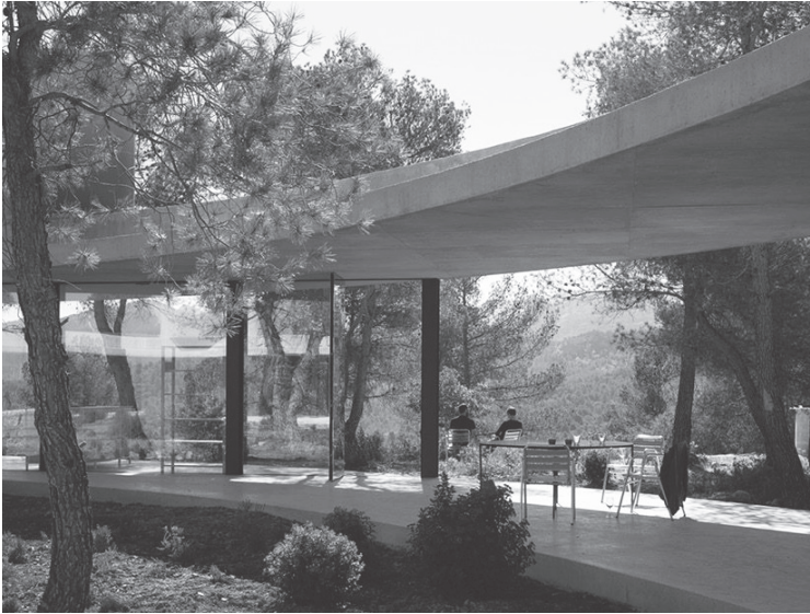
Fig.42 Office, Solo house, 2012-2017. «The roof functions as a shelter, and forms the perimeter of the inhabited surface. It is supported by four straight rows of eight columns, which cut chords from the circular base shape. Only these four areas are inhabited, with variable levels of protection. Large stretches of curtain facade slide on the outer edge of the circle, allowing the living areas to fully open, and providing a maximum relationship between the dweller and the surrounding nature.» Description des architectes
