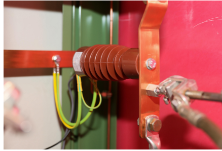
Figure 4.10 – 18-kV voltage transducer installed in the primary substation of a medium voltage distribution network (courtesy of Murielle Gerber, EPFL). The distribution network was employed in the pilot test of EMTR-based fault location methods.
