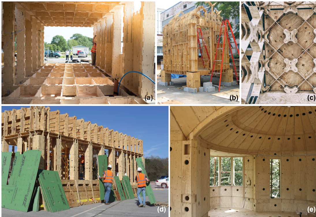
Figure 3.4 – (a) WikiHouse [165] / (b) Wood Frame Grammar system [133] / (c) X-Frame system [168] / (d) Sim[PLY] system [149] / (e) Facit Homes system [40].
