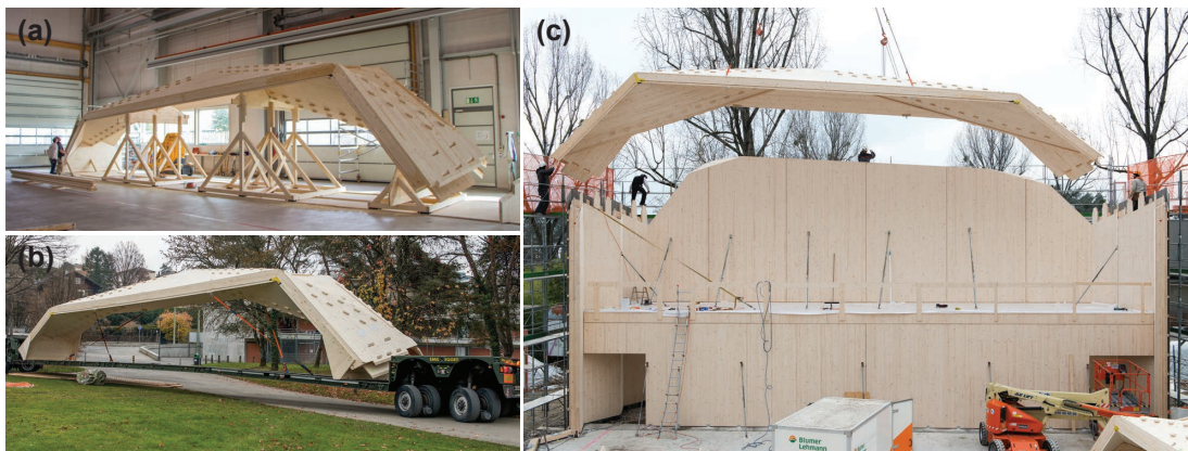
Figure 2.4 – Photographs of the construction system process: (a) Prefabrication of a roof element / (b) Transport of a roof element / (c) Onsite assembly of the roof and wall elements.
