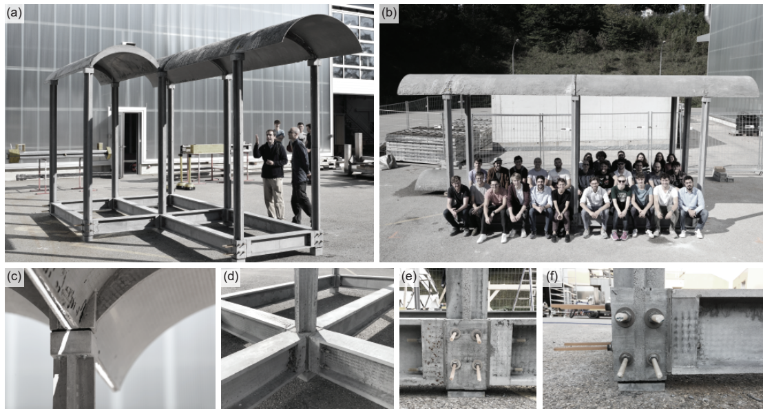
Figure 4.11: Final structure: (a) three modules; (b) construction staff; (c) column-head connection; (d-f) connections of the base frame.
