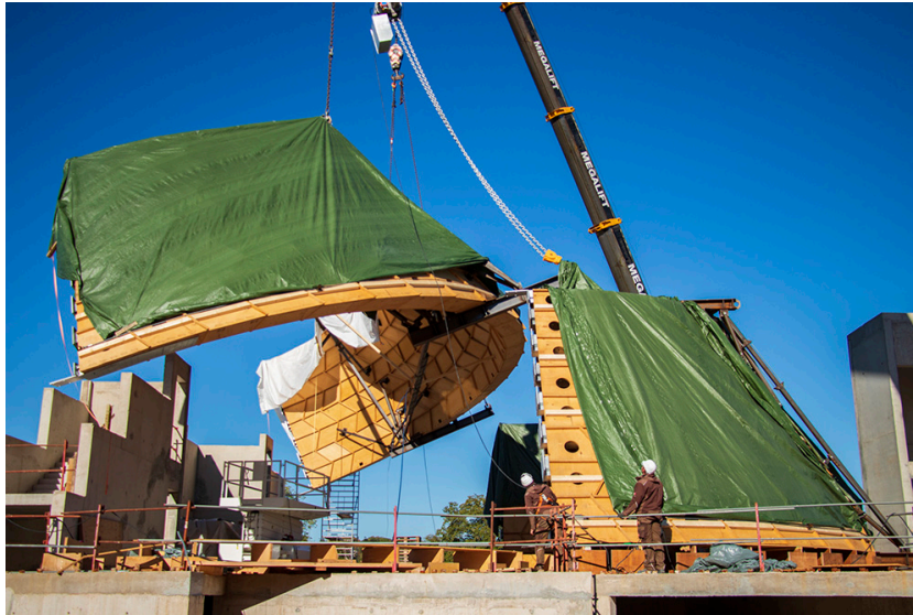
Figure 1.14 – Assembly of the Annen Plus SA head office arches. Structures assembled lying on their longitudinal side are positioned by lifting them up with a crane in one single assembly. © 2019 Annen Plus SA.
