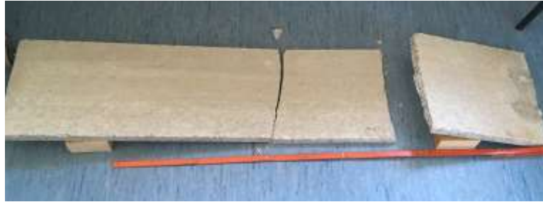
Figure 8: Unexpected damage on reused component in K.118 (Baubüro in situ, 2018)
