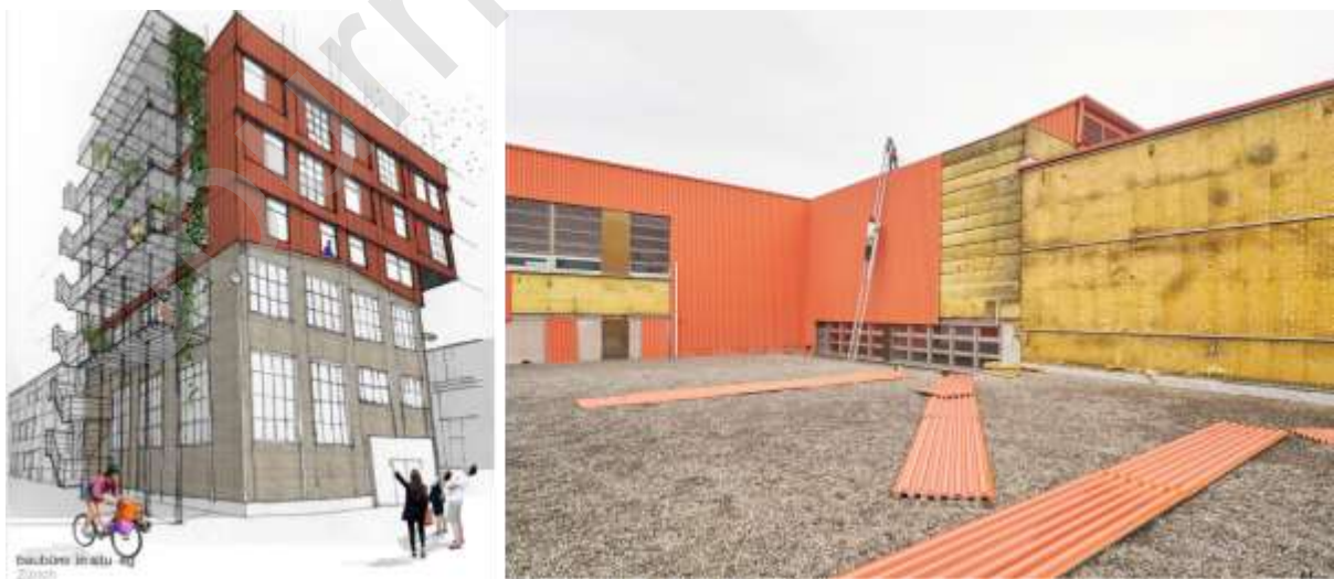
Figure 3: Design of K.118 and dismantling of façade elements leading to the choice of the red colour for the façade (Baubüro in situ, 2018)
