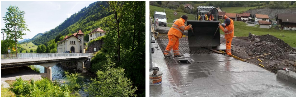
Figure 11. Montbovon Bridge after strengthening and rehabilitation, and UHPFRC casting.
