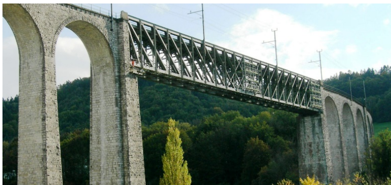
Figure 4. Railway bridge across the River Rhine at Eglisau, Switzerland.
