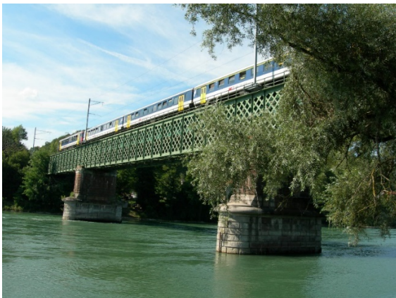
Figure 1. The railway bridge over the Rhine River between Koblenz (Switzerland) and Waldshut (Germany) is in service since 1859. Its performance in terms of fatigue and structural capacity is sufficient to fulfill the requirements of future rail traffic of higher demand (Brühwiler 2012). After the execution of low-cost maintenance interventions, the bridge now has a low “equivalent age”.
