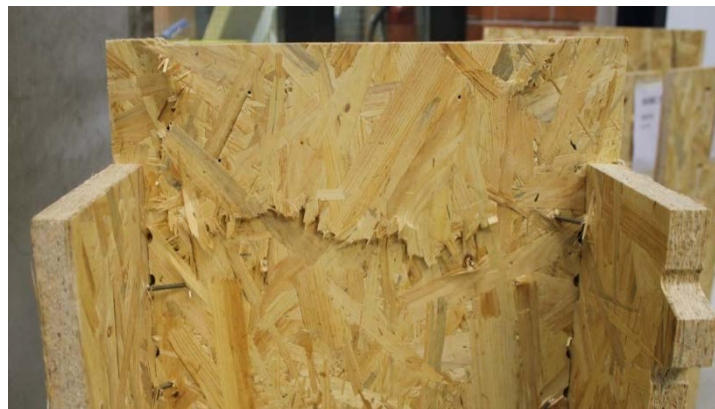
Figure 15: Failure of the web
