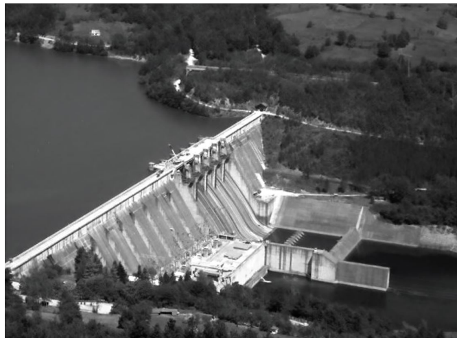
Figure 1.1 – Bajina Basta dam, Serbia. Spillway consisting of a gated ogee crest followed by a smooth chute with energy dissipation in a stilling basin.
