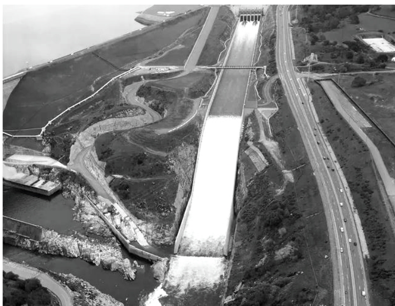
Figure 2.21 – Folsom dam with auxiliary stepped spillway, USA. Photo from https://kfbk.heart.com/featured/cristina-mendonsa/content/2019-02-13-making-room-for-the-pineapple-express/ .
