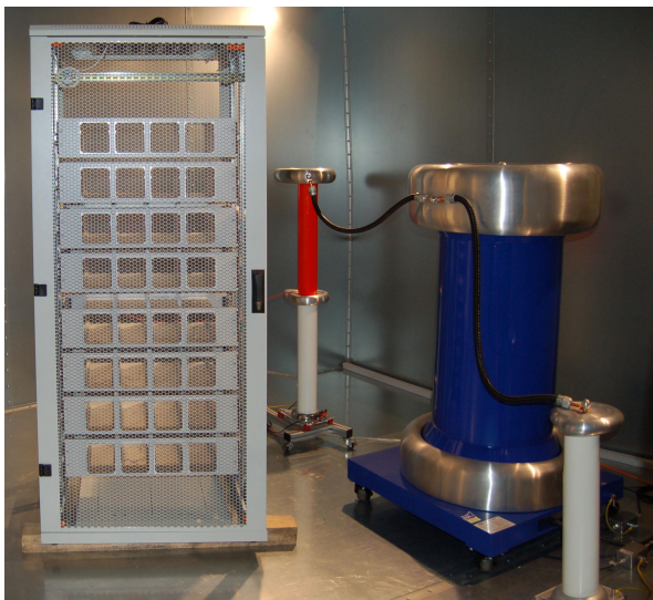
▲ Cabinet of one phase-leg (32 cells) in Faraday cage during insulation coordination testing
