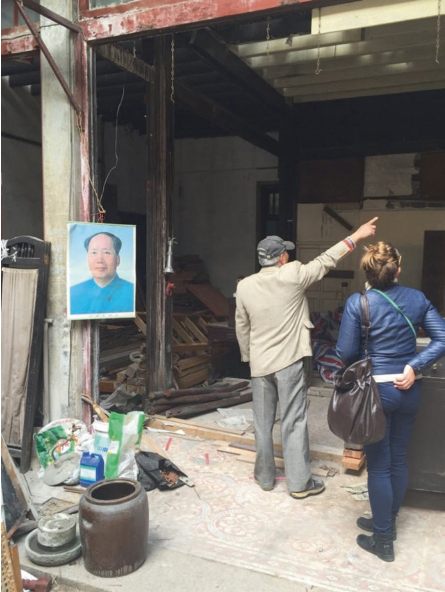
Fig. 3.1 Destruction for renovation in downtown Shanghai 2014. (Reproduced with permission from Boley)
