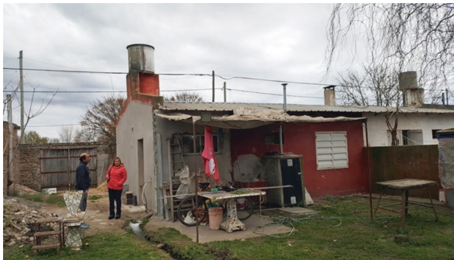
Fig. 6.14 Barrios Unidos: rehabilitation of a house in a social housing development Argentina. (Reproduced from Vexina Wilkinson 2017)
