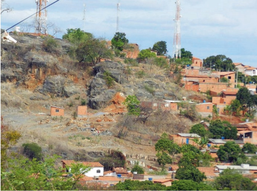
Fig. 5.19 Recent constructions in the hills near Montes Claros in 2015. (Reproduced with permission from Bolay)
