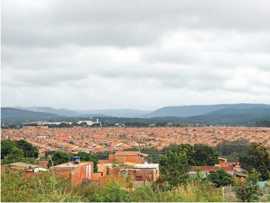
Fig. 5.15 New social housing in the outskirts of Montes Claros in 2018. (Reproduced with permission from Bolay)
