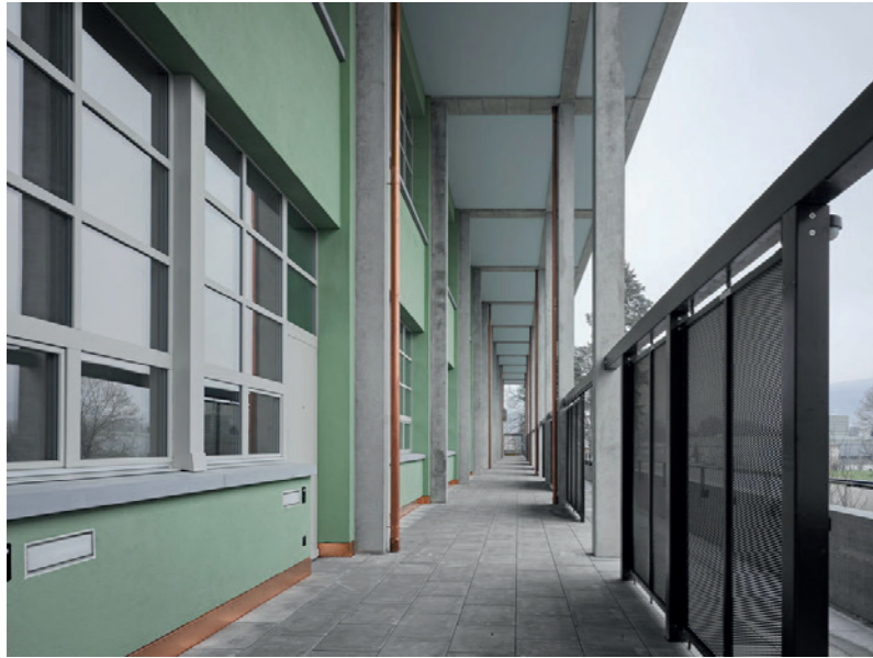
Terrasses privatives, coursives, façade Nord ( http://www.adrianstreich.ch )
