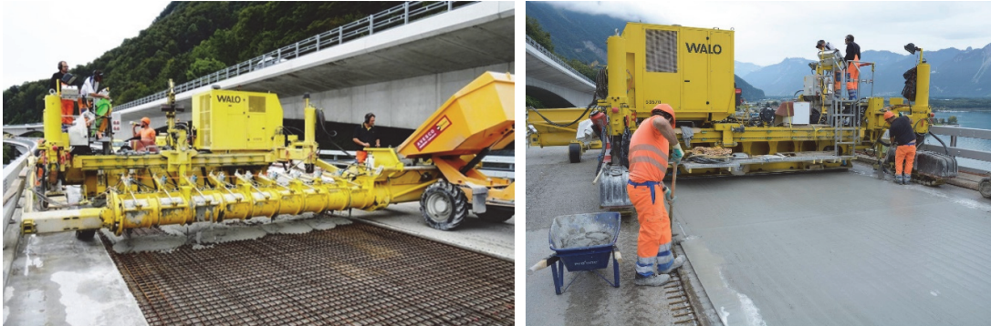
Fig. 2_ Strengthening of the Chillon viaducts with R-UHPFRC (photos from [16])
