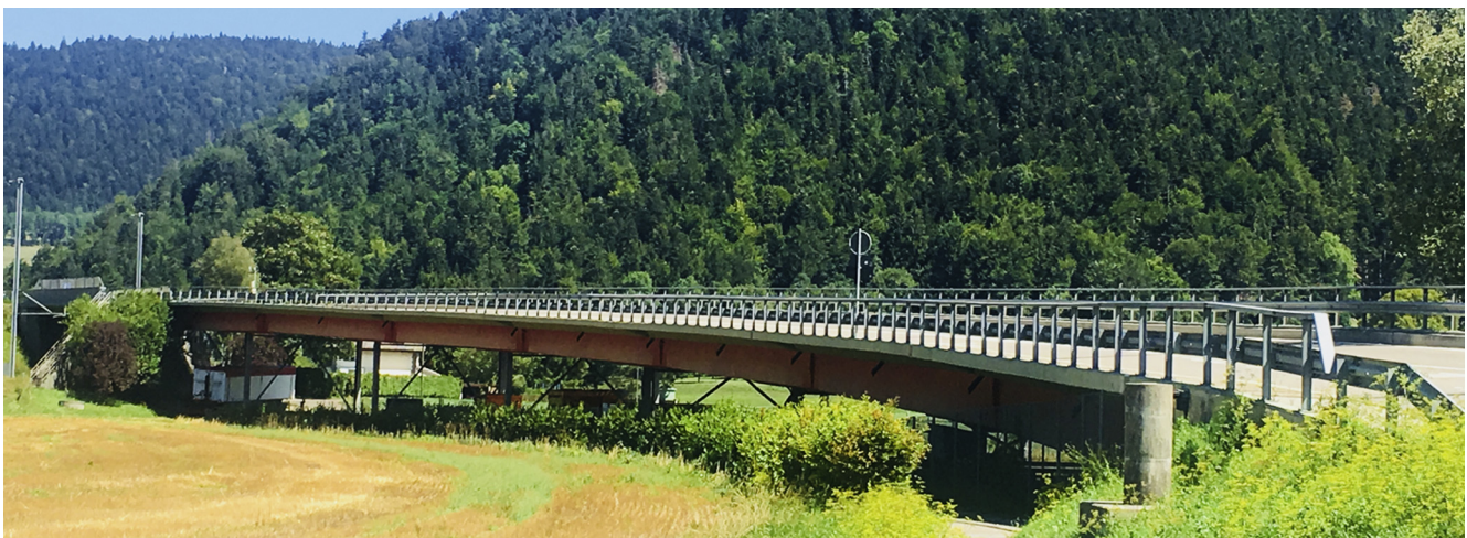
Fig. 1. View of the investigated steel-concrete composite viaduct.
