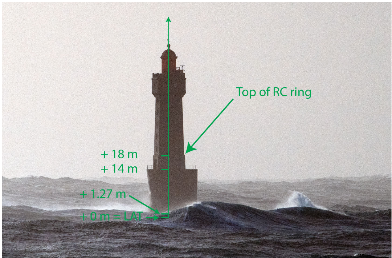
Figure 9. Reference picture from series 1, without breaking wave [45], 1 minute before wave1 hit the lighthouse.
