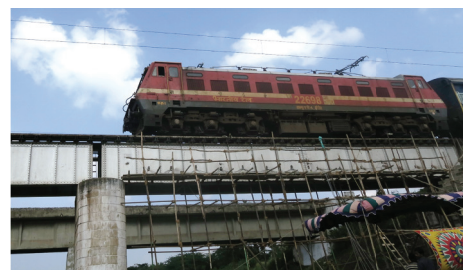
(b) Instrumented bridge (Ponneri)
