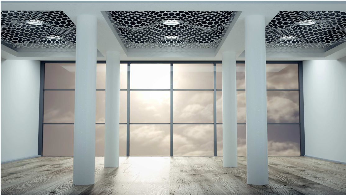
Figure 5.3 – Interior decorative cladding. This hanging structure has been optimized to align with the boundary constraints imposed by the ambient space. The designer controls the shape by interactively modifying scale factors while allowing the triangles to slide along the boundary curves.
