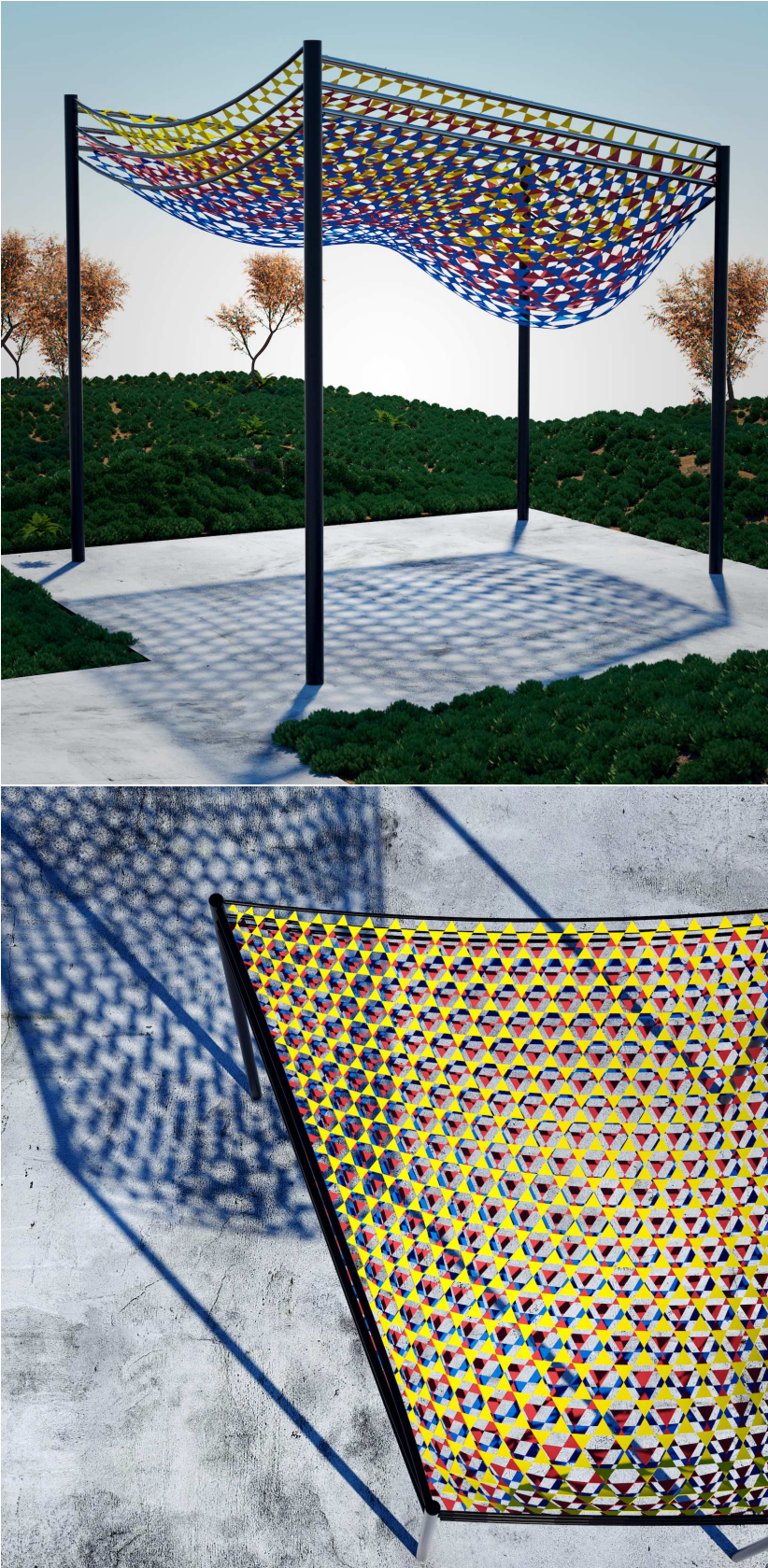
Figure 5.4 – Multi-layer shading pavilion deployed by gravity.
