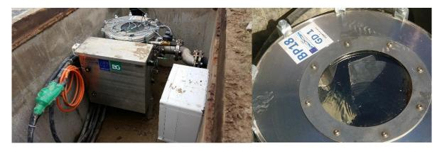
Figure 2: Installed prototype sealed vortex siphon (courtesy of BG)
