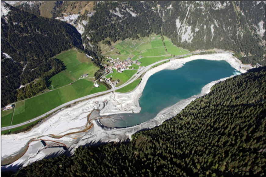
Fig. 73.1 Sedimentation of Sufers reservoir, Grisons, Switzerland
