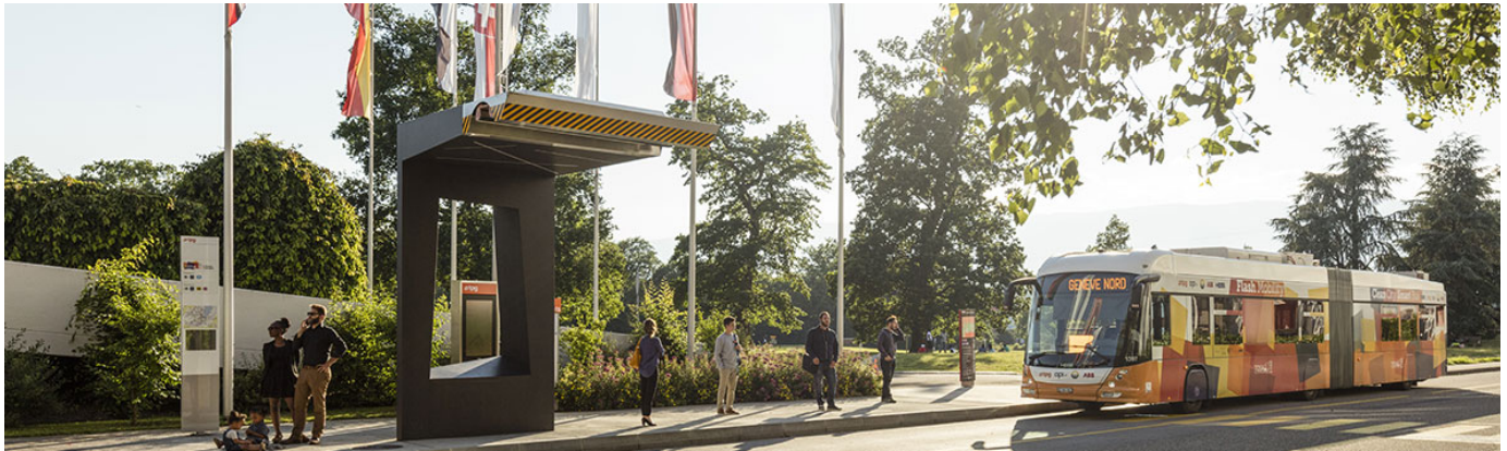
▲ TOSA flash charging e-bus (Source: https://new.abb.com/substations/references-selector/tosa-flash-charging-e-bus-geneva-switzerland )
