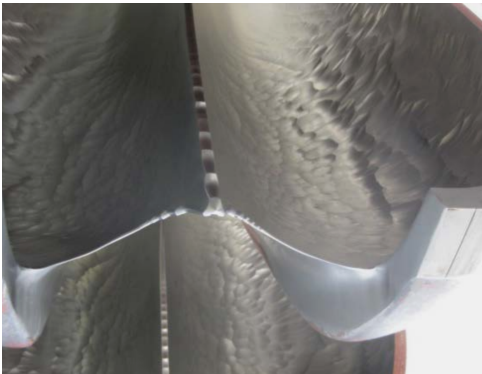
(c) Uncoated bucket at the Emosson power plant [50].
