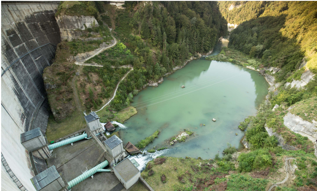
Figure B.2 – Stilling basin of the Rossens Dam and the begin of the residual flow segment in a narrow valley (wetted width 20-30 m). Image taken on 13 September 2016, courtesy Research unit Ecohydrology, ZHAW
