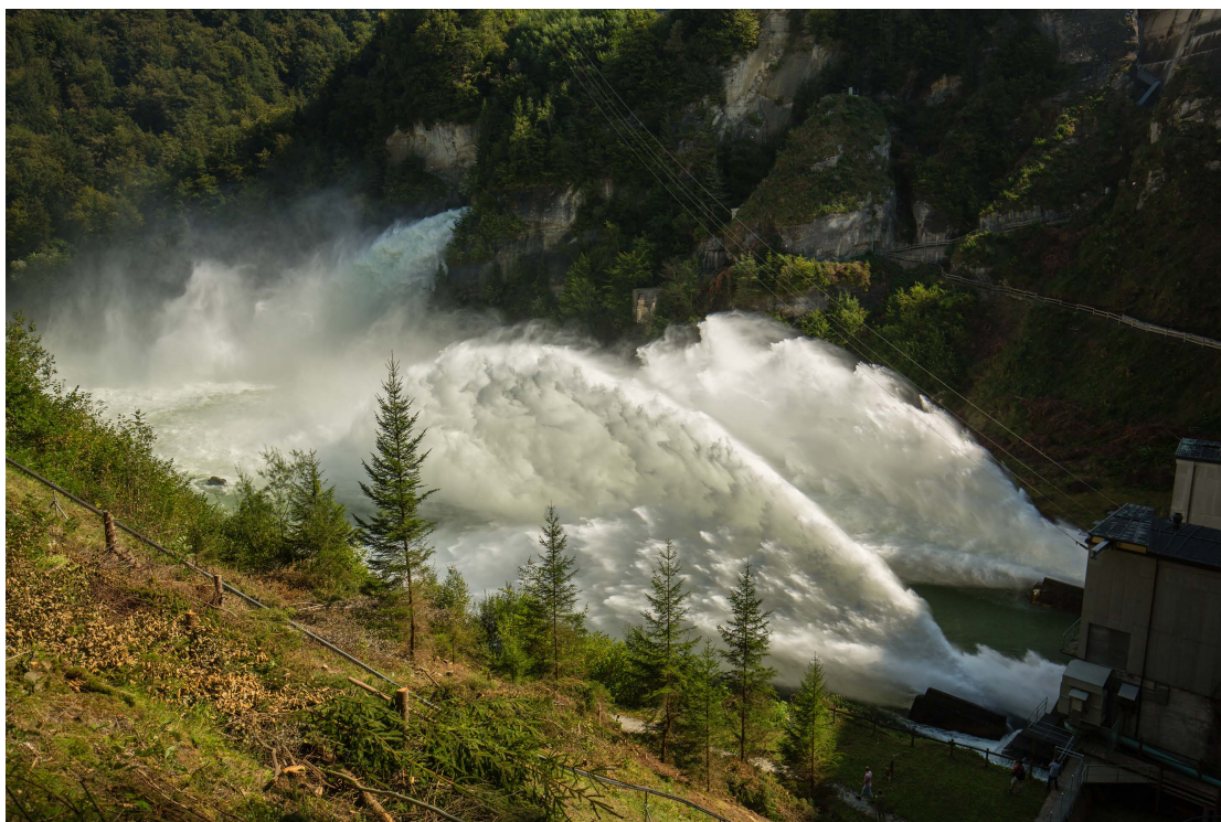
Figure E.1 – Bottom outlet of the Rossens Dam during the artificial flood in the Sarine River on 14 September 2016. Image courtesy Research unit Ecohydrology, ZHAW
