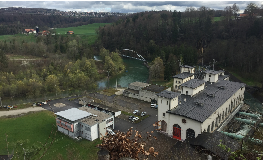
Figure B.5 – Turbine house in Hauterive, Fribourg, is located in a sharp left bend of the Sarine. Up to 75 \text{ m}^3 \text{ s}^{-1} are released by the four Francis turbines. The four restitution tunnels can be seen right of the turbine house, the restitution channel enters the Sarine below the pedestrian bridge in the center of the image. Image taken on 11 April 2016, courtesy Severin Stähly
