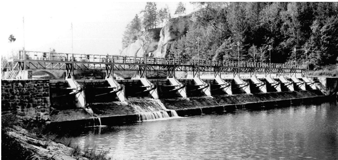
Figure 3.4 – Water intake of the former Thusy-Hauterive hydropower plant. The weir with 12 segment gates diverted the water from the Sarine through a tunnel to the powerplant in Hauterive from 1902. The Thusy water intake and its famous bridge in the back are inundated by the Lac de la Gruyère today. Image courtesy Bibliothèque cantonale et universitaire Fribourg. Fonds Mülhauser
