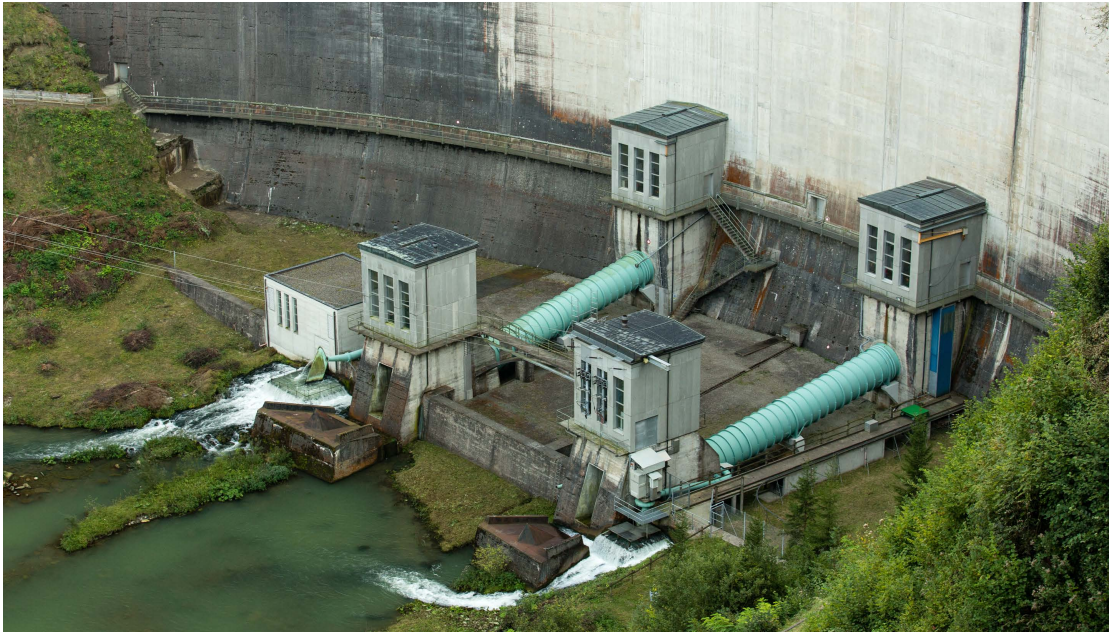
Figure B.1 – Bottom outlets of Rossens Dam with residual flow turbine producing 13.6 GWh per year. Image taken on 13 September 2016. Image courtesy Research unit Ecohydrology, ZHAW
