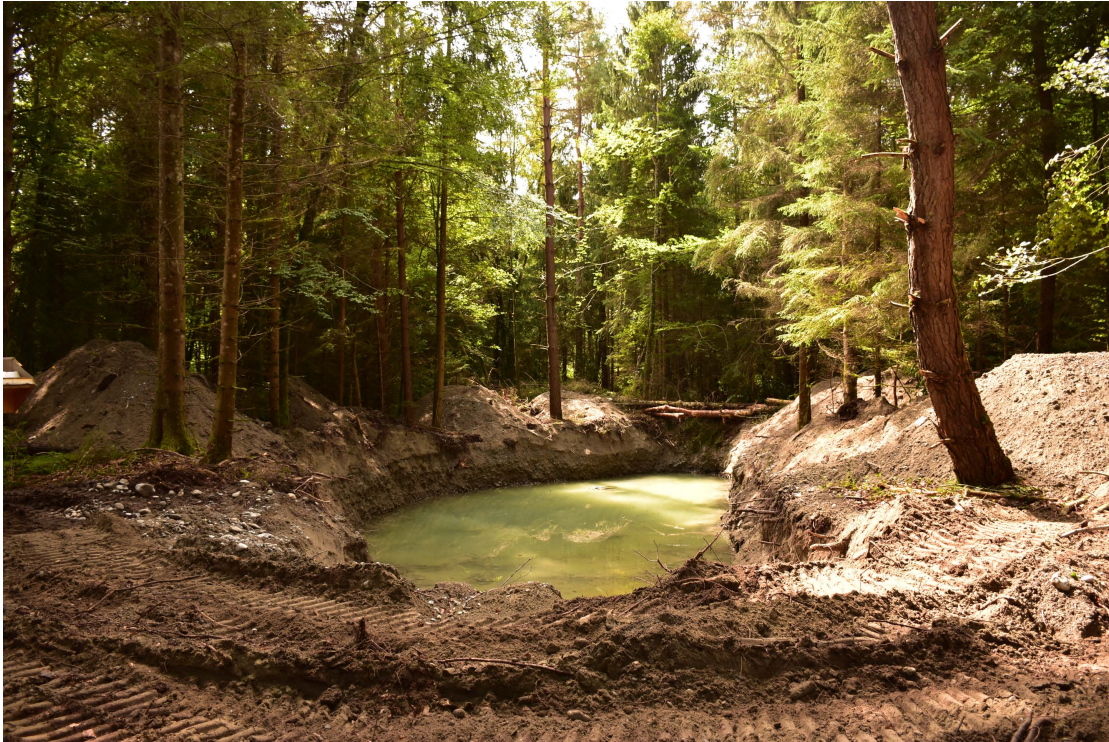
Figure D.1 – Excavation resulting from the sediment replenishment in the adjacent alluvial forest. Groundwater infiltration created a pond which serves as new created habitat in the floodplain and only meters away from the river channel. Image courtesy Elena Battisacco
