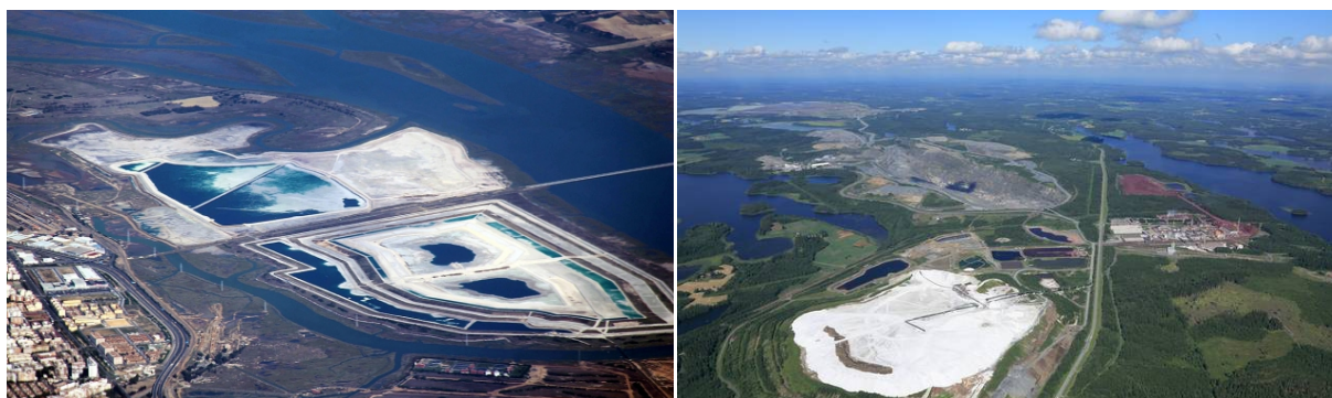
Figure 22-1: Deposits of phosphogypsum: at Huelva, Spain, covering ~ 1200 ha (left) 27 and near Siilinjärvi, Finland, covering ~ 60 ha (right) 28 .
