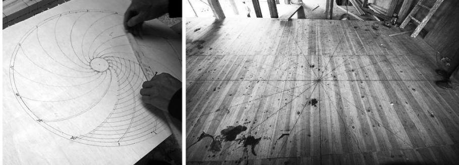
Figure 4. left: Master Liqun Zhang demonstrated the sketch of a new-built spiral zaojing on site, the scale of 1:10. Ref. ZJ-04; right: Master Shichun Wang demonstrated the sketch of a new-built spiral zaojing on the floor on site, the scale of 1:1. Photo: Lijia Wang.
