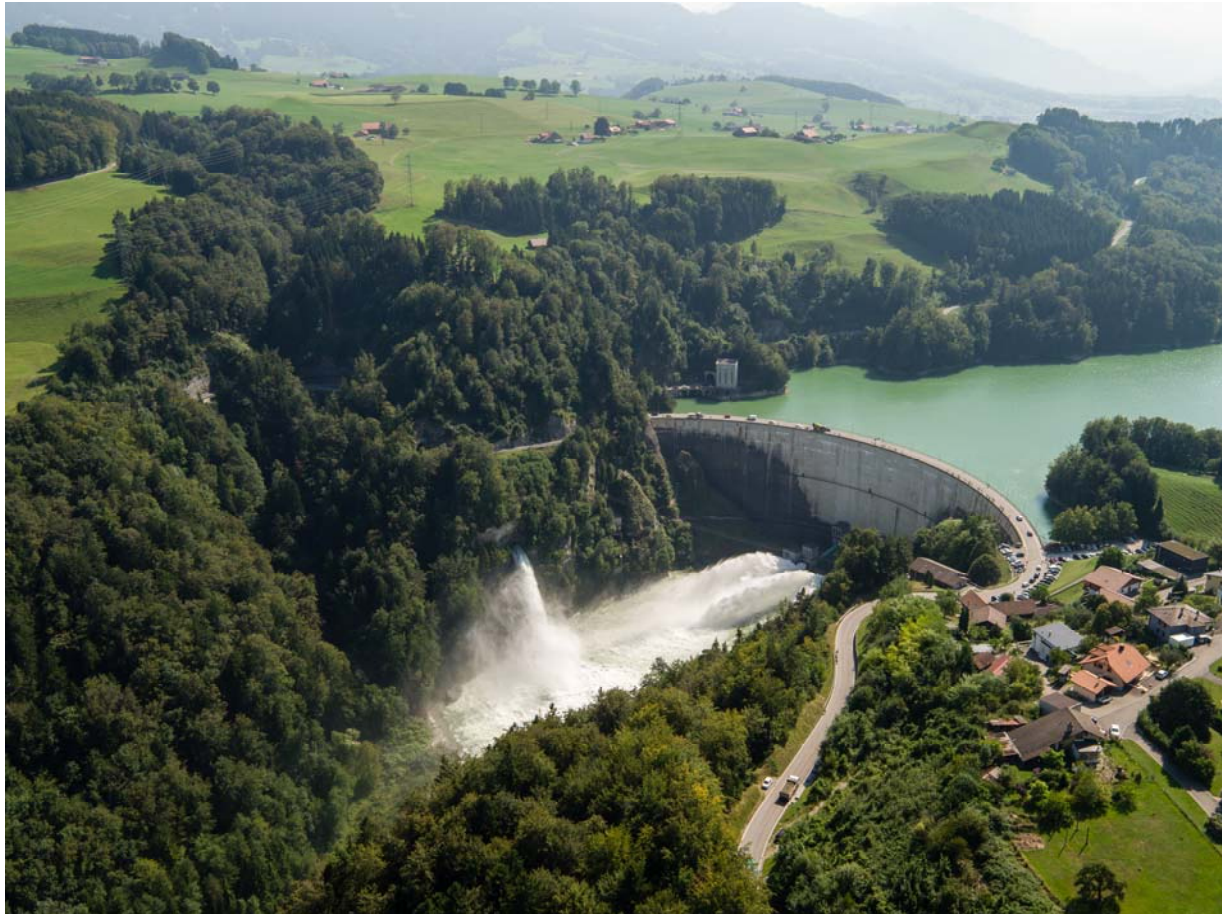
Fig. 3. Air-view of the Rossens dam during the release of the artificial flood on 14 September 2016. Image © Research Unit Ecohydrology, ZHAW
