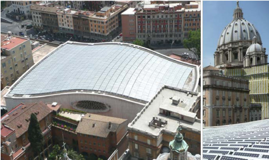
PV system on the roof of Aula Pierluigi Nervi Vatican City.
