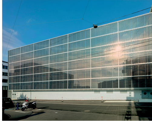
(b) Façade PV installation
