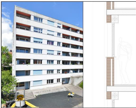
Figure 1: Scenario E0 - Current Status. Image and construction detail of the existing façade.
