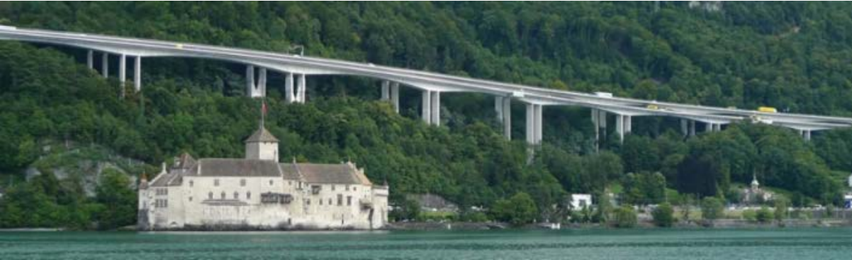
Figure 6. Chillon Viaducts along Lake Geneva.
