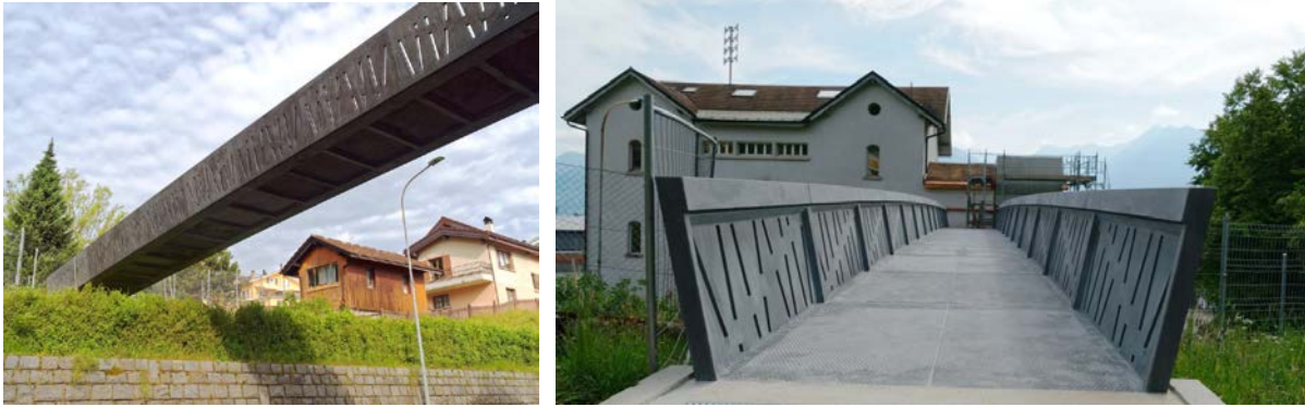
Figure 13. Footbridge at Le Bouveret: 25m span girder spanning over a road (left); symmetric cross section with inclined webs (right), before opening in June 2018.
