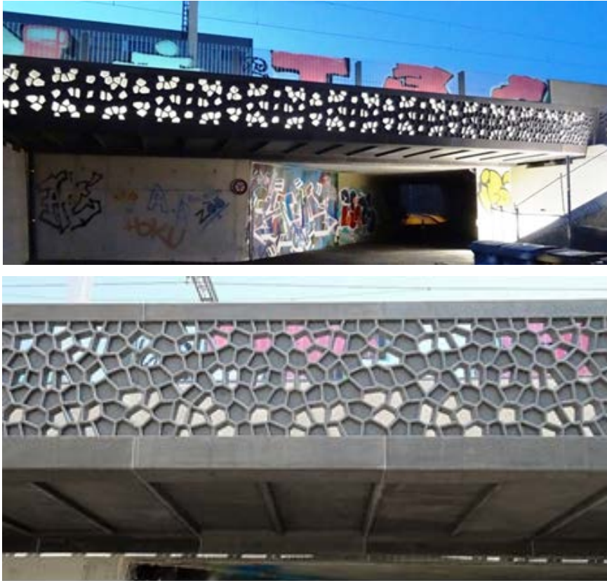
Figure 11. Martinet Footbridge: view of illuminated bridge at dusk, after opening in July 2015 (left), and view of the “organic” web and underside of the ribbed slab (right).
