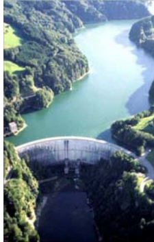
a) Rossens dam
