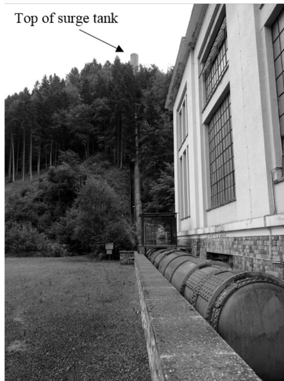
Figure 1.4 – View of the Wevercé (Eastern Belgium) surge tank from the powerhouse
