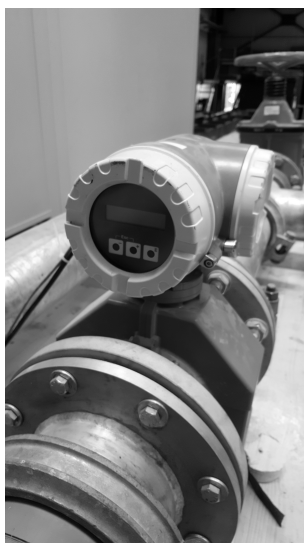
Figure 4.9 – ENDRES + HAUSER - PROMAG 50 W flowmeter
