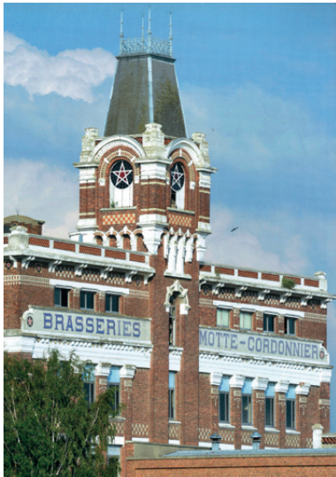
Fig.6. Usine Motte Cordonnier
